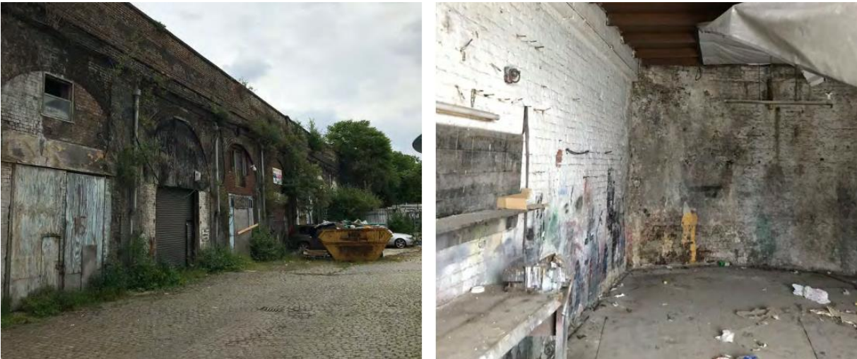
Image 3.8: View of railway arches external and internal
